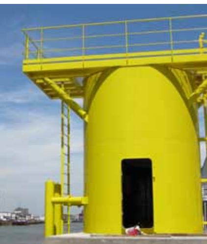
Wind turbine foundation installation
