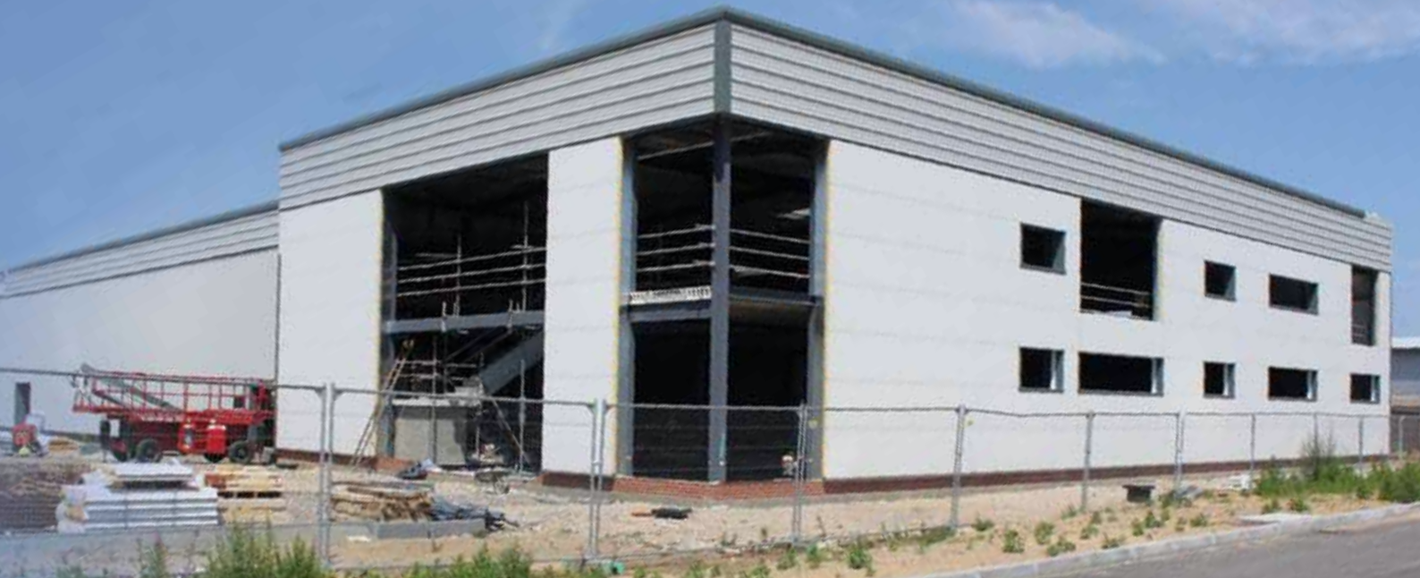
Construction on new NCL factory at Beacon Park
